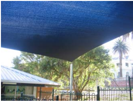
Kindergarten Shade Area
